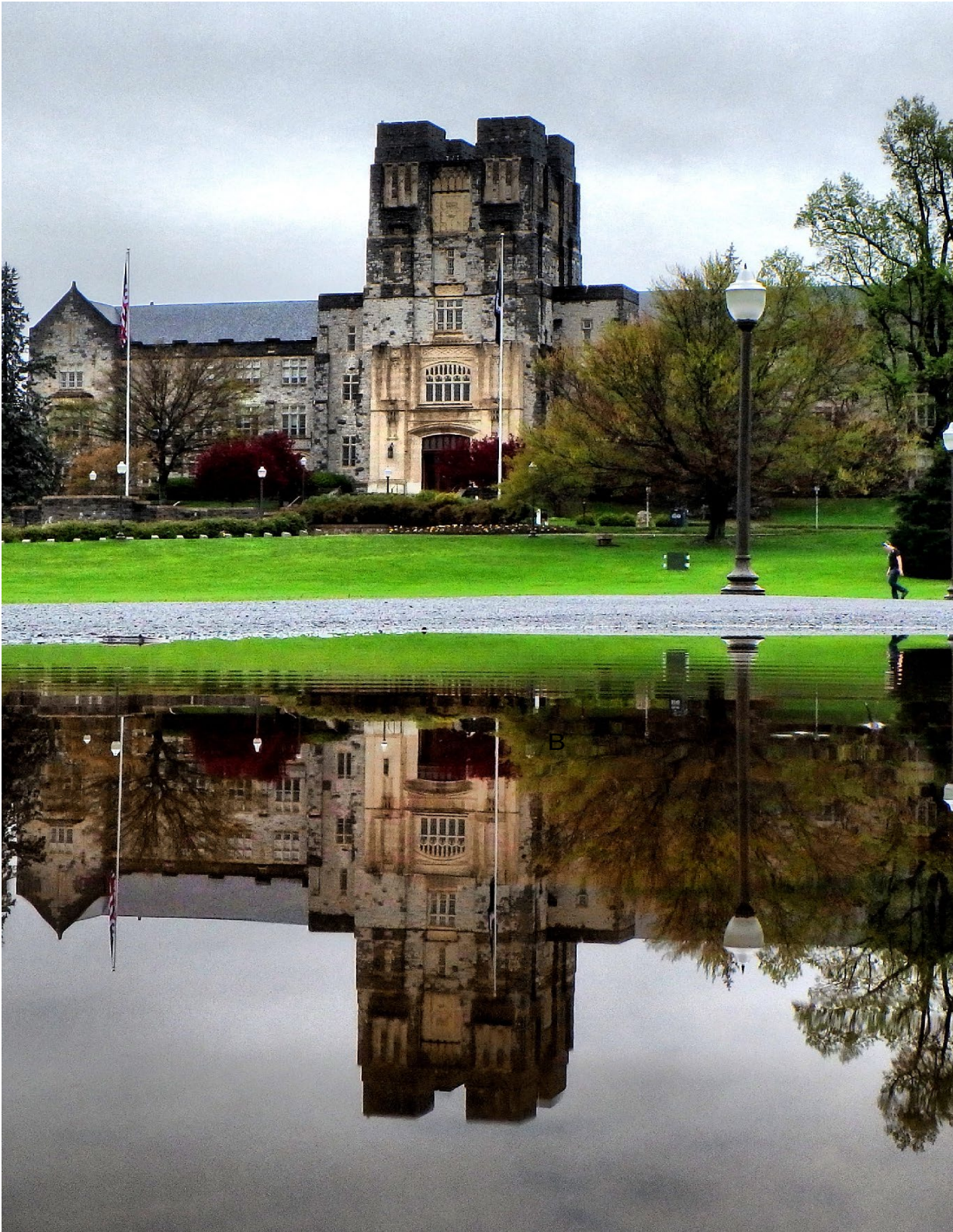
Burruss Hall, Flooded Drillfield
